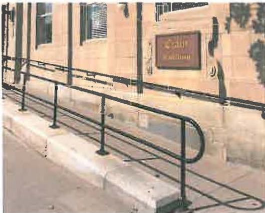
Figure 3.0: Accessibility ramps ensure that entrances to businesses are barrier-free – Perth, Ontario.
